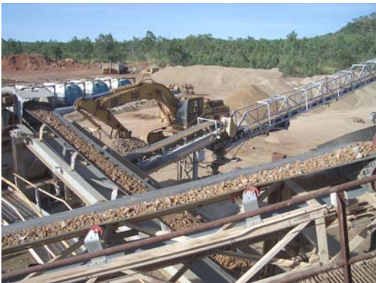
Crushing stockpiled inventory – April 2008
